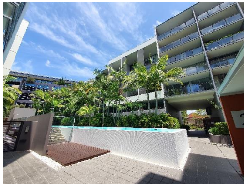
Figure 11 2-4 Powell Street internal courtyard and pool (isolated from Powell Street)
