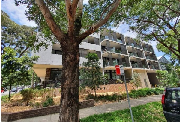
Figure 4 10-20 McEvoy Street Residential Complex facing South
