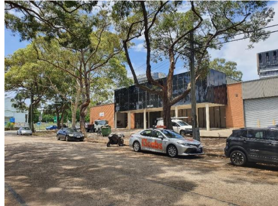
Figure 7 267 Young Street facing North-East
